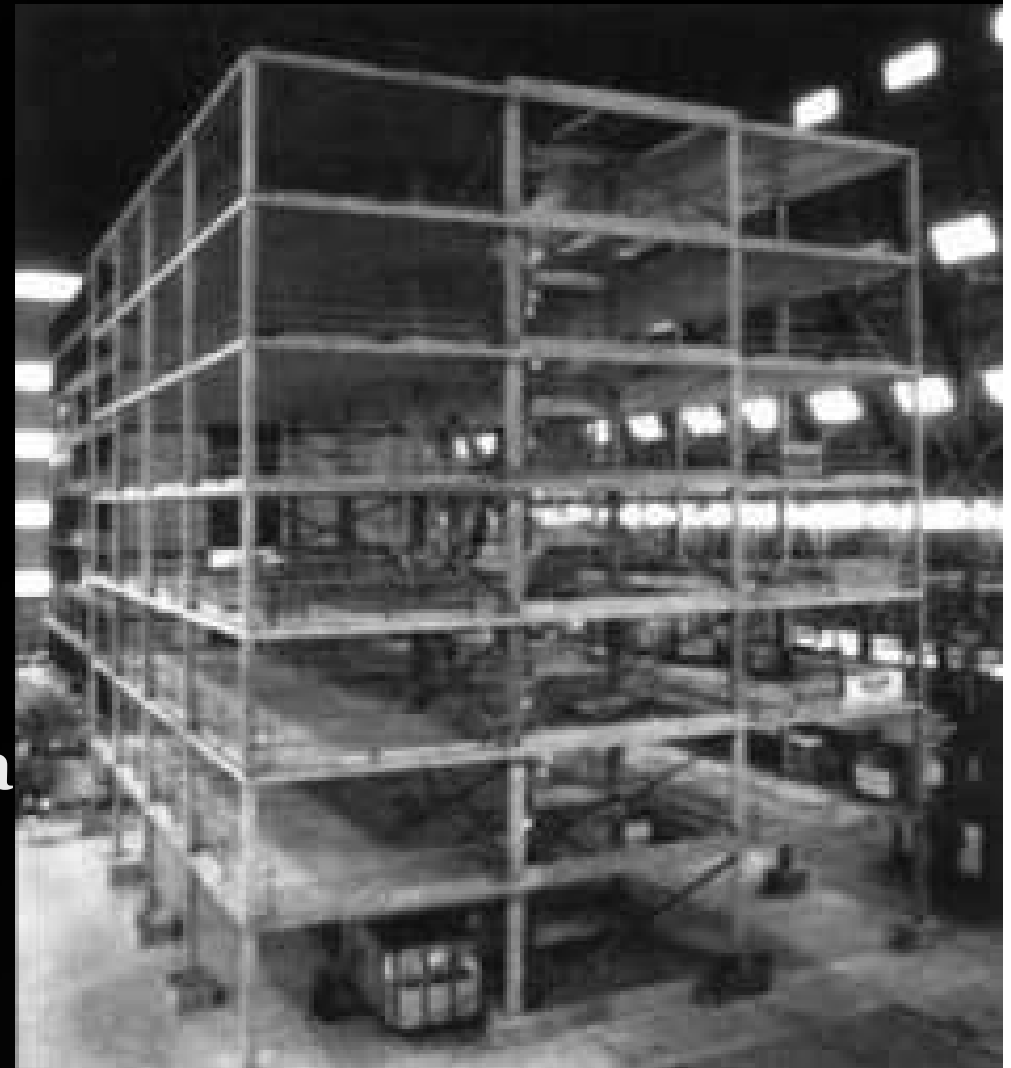
Cardington Concrete Building Frame
