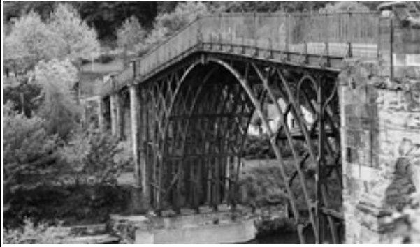
Primer Puente Metálica → 1779 d.C. Coalbrookdale Bridge in Telford, Inglaterra still in use today carrying occasional light transport and pedestrians
