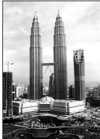
Petronas Towers Cesar Pelli Kuala Lumpur Malasia 1.997 452m f_{ck} = 80 \text{ MPa} before / after
