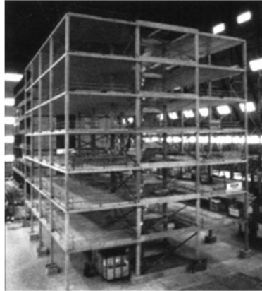
Cardington Concrete Building Frame
