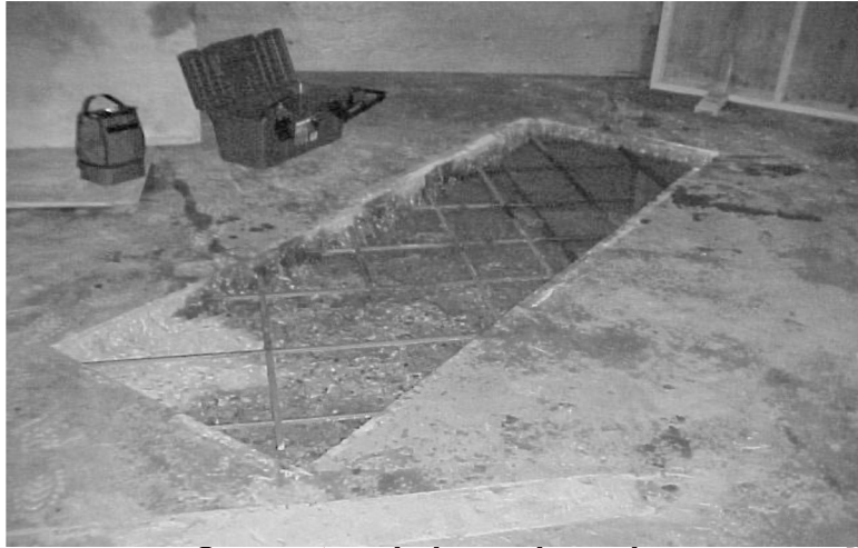
Saw cut and cleaned repair area.
