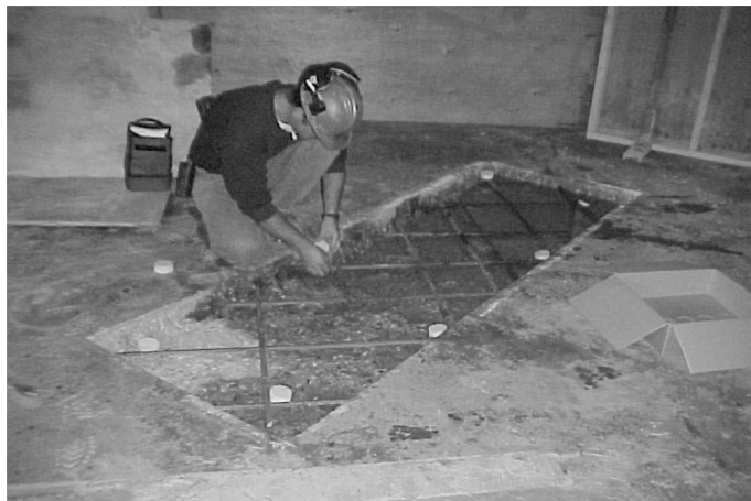
Installing anodes around the perimeter of the repair.
