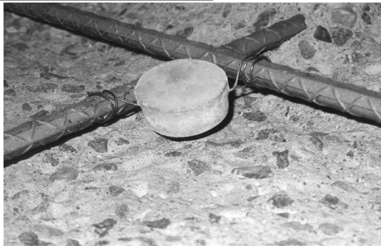
Anode is tied to reinforcing steel quickly and easily.
