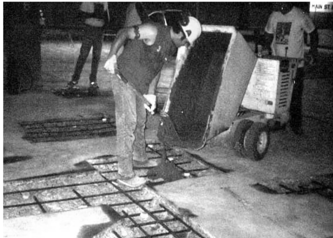
Embedding anodes with repair material.
