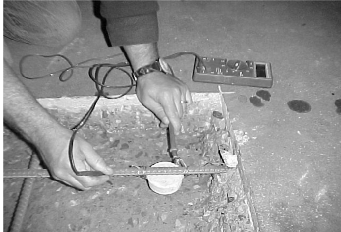
Testing anode connection to reinforcing steel.
