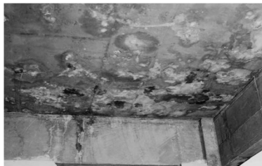
Fig. 39 Cracking and Upheaving of a Tile Floor Due to Sulphate Action in Base Concrete C. D. R. AGGARWAL
