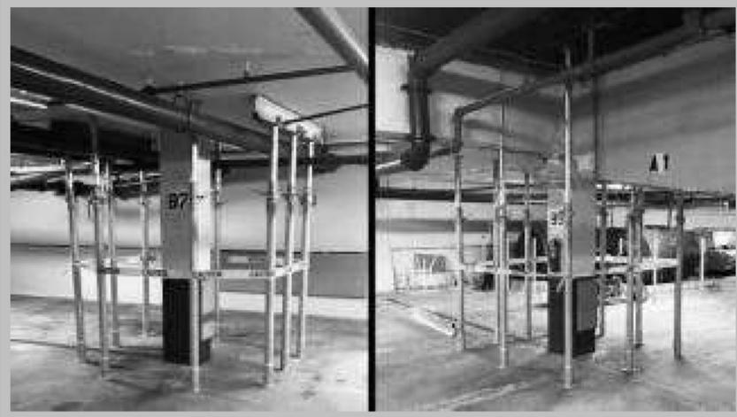
Shoring is visible around at least 11 columns at Champlain Towers North, sister building to the Champlain Towers South condo that collapsed in June 2021.
