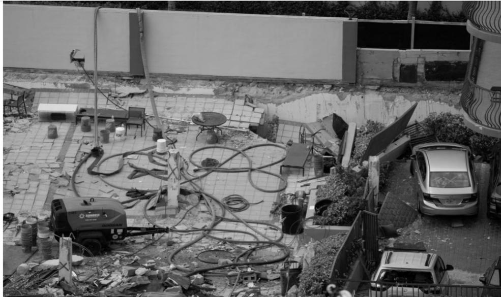
A photo of the Champlain Towers South pool deck shows the slab disconnected from the southern wall during the June 24 collapse. Damage in the failure plain is not uniform, indicating pre-existing damage to portions of the slab at the connection, according to engineer Dawn Lehman. Robert Lisman
