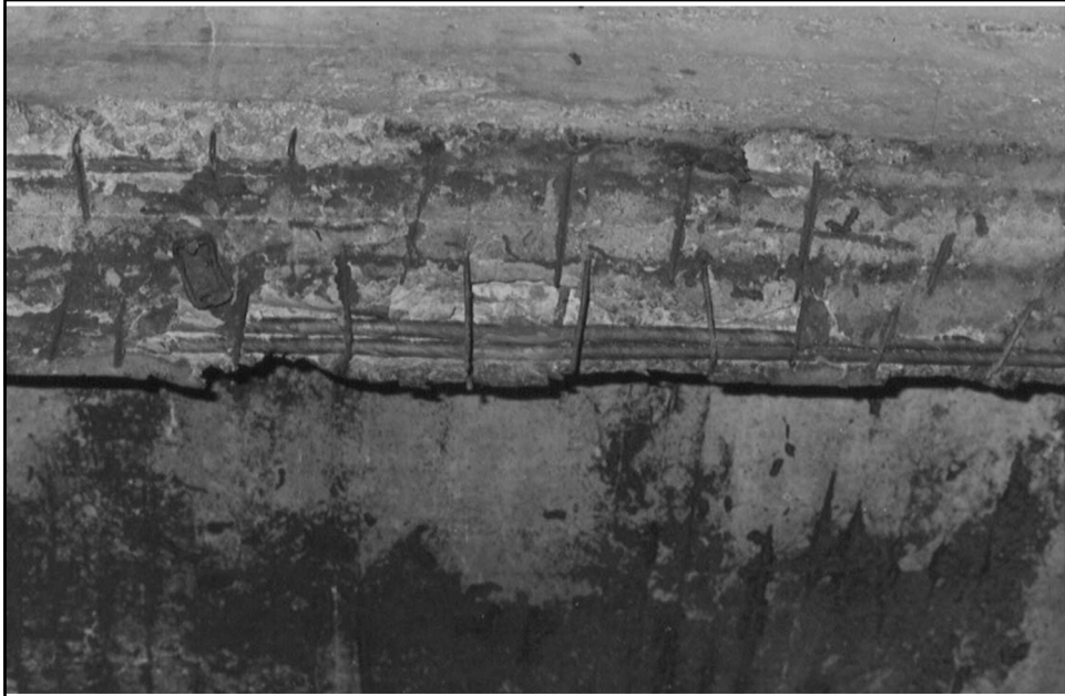
typical beams aspect
