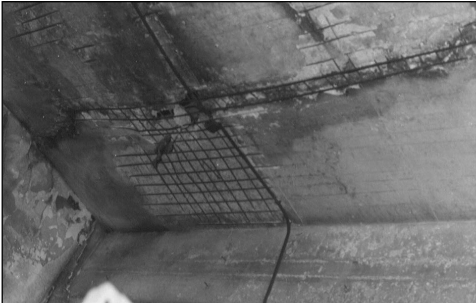
typical slabs aspect
