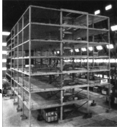
Cardington Concrete Building Frame
