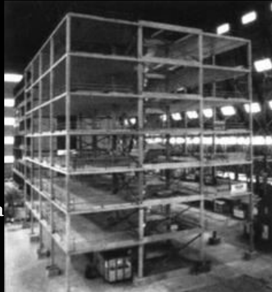
Cardington Concrete Building Frame
