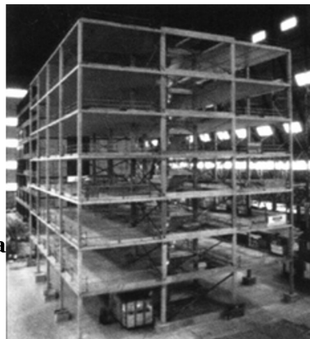
Cardington Concrete Building Frame
