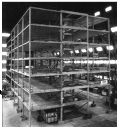
Cardington Concrete Building Frame
