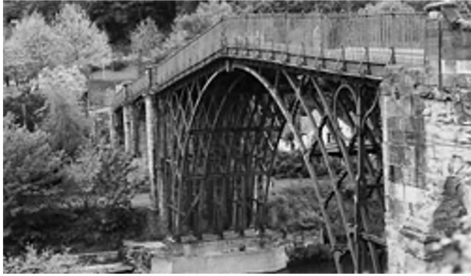
Primeira Ponte Metálica → 1.779 d.C. Coalbrookdale Bridge in Telford, Inglaterra still in use today carrying occasional light transport and pedestrians
