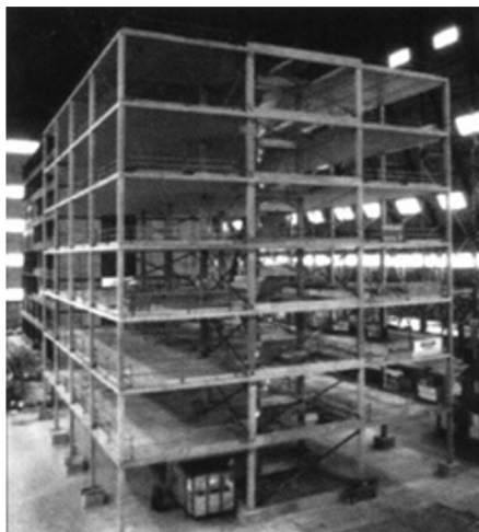
Cardington Concrete Building Frame
