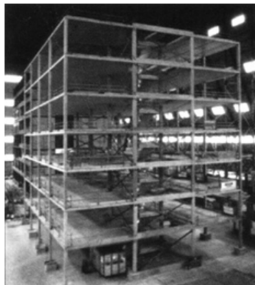
Cardington Concrete Building Frame
