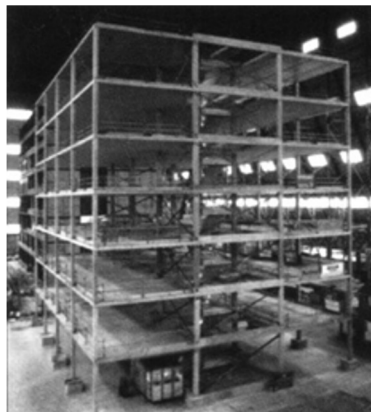
Cardington Concrete Building Frame
