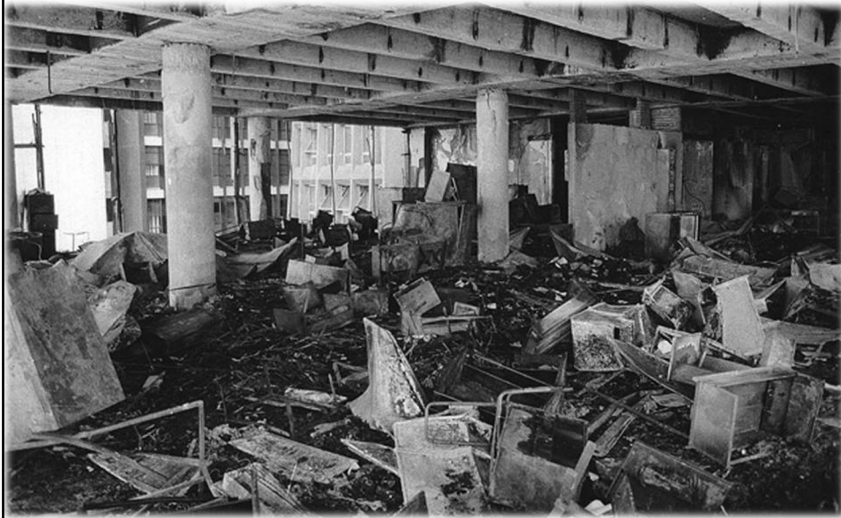
Ribbed slab with band beams
