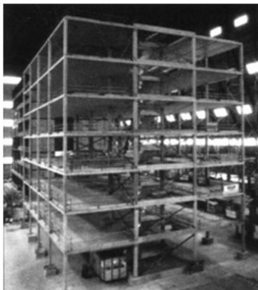
Cardington Concrete Building Frame
