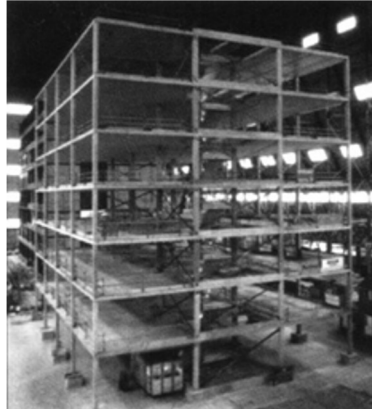
Cardington Concrete Building Frame
