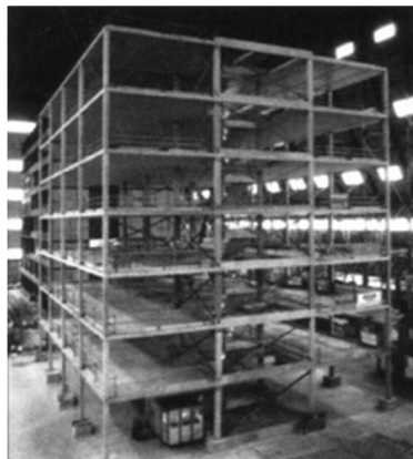
Cardington Concrete Building Frame
