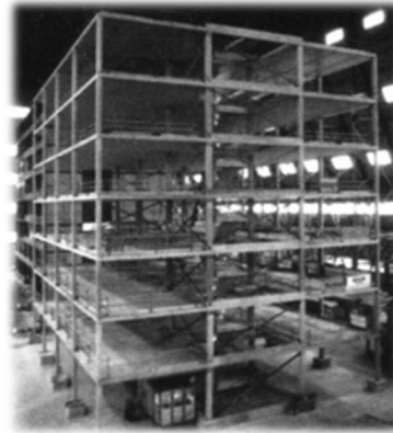
Cardington Concrete Building Frame
