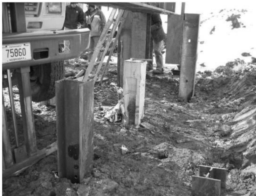
Figure 22. Photo. Experimental precast pile made of UHPC
