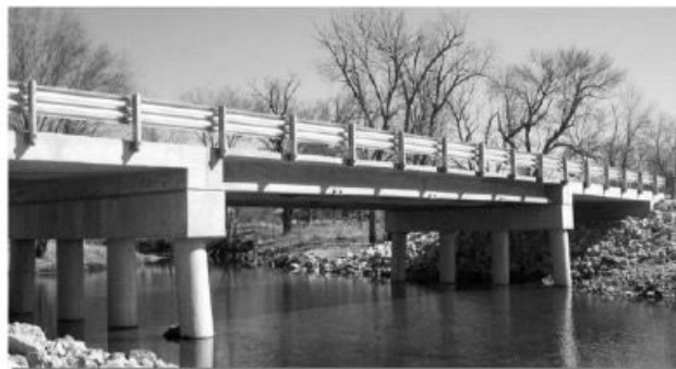
Figure 15. Photo. Jakway Park Bridge, Buchanan County, IA
